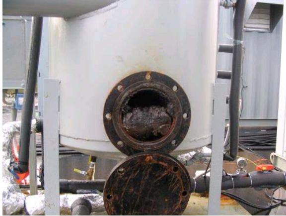
Figure 3. Solid NAPL in the Bottom of the Vapor/Liquid Separator
