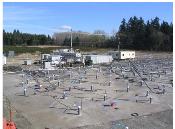
Figure 2. ERH Equipment & Electrode Layout in NAPL Area 2
